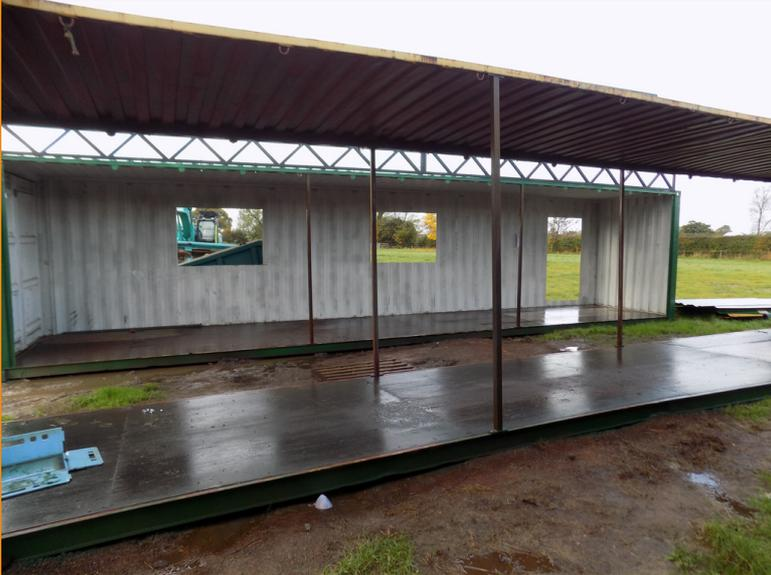
The rear door and back window apertures have been cut, and will be reinforced with welded steel frames.
